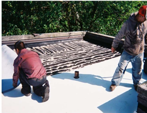
Roll UltraPly TPO XR into XR Stick or ISO Spray R Adhesive
