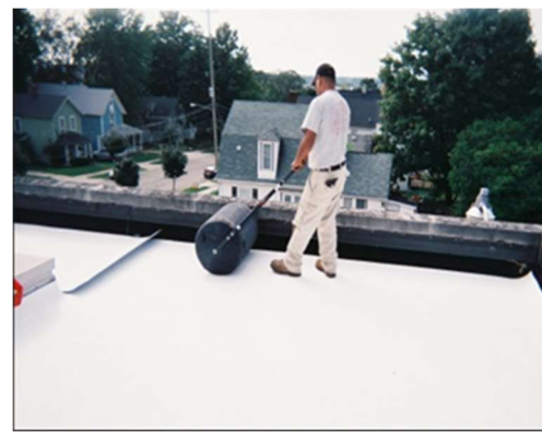
Apply pressure to the top surface of the membrane to ensure contact with a roller (not to exceed 150 lb/68 kg)
