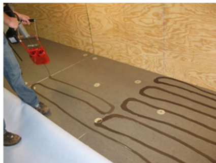
Bead application of XR Stick in cartridge on mechanically attached Polyisocyanurate insulation board @ 6" o.c.
