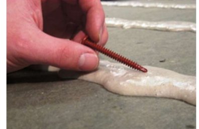
STEP 3: Tack-free stage – ready for application of UltraPly TPO XR Membrane (after 5 - 7 minutes)
